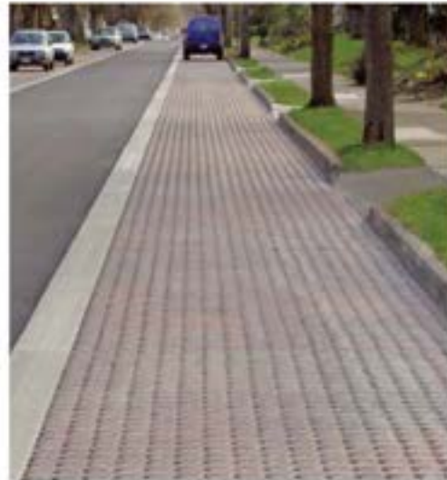
Figure 18 - The completed permeable pavement at Westmoreland Neighborhood
