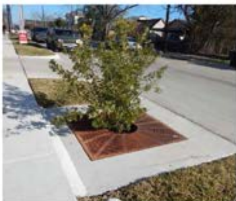
Figure 8 - Completed tree box Photo courtesy of and copyright Watearth, Inc.
