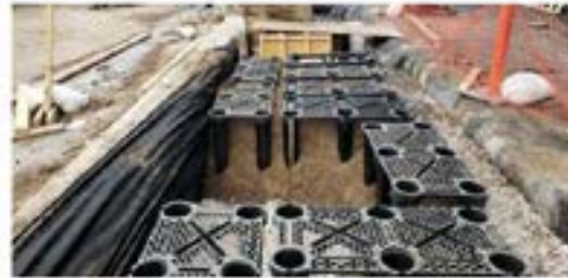
Figure 7 - The Silva cell suspends pavement and allows for more soil volume and loosely compacted soil.
