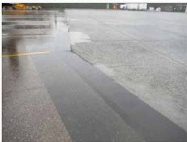
Figure 14 - Permeable pavement post-installation Photo courtesy and copyright of Watearth, Inc.
