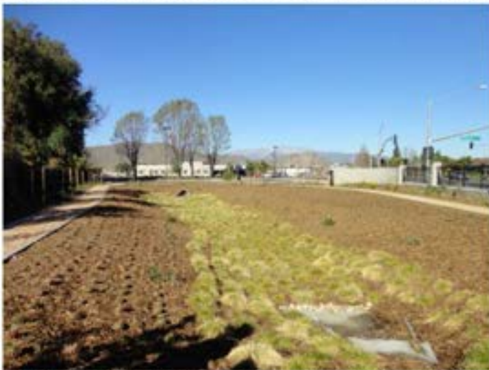
Figure 3: Vegetated Swale Example – Riverside County Flood Control District, California Photo courtesy of and copyright, Watearth, Inc.
