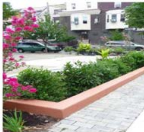
Figure 11 - Planter box in Columbus Square 0.74 acre-inches of runoff from every storm
