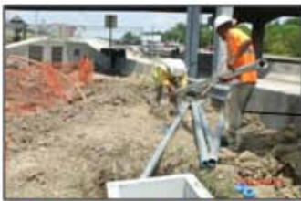
Connecting the Rigid Metal Conduit
