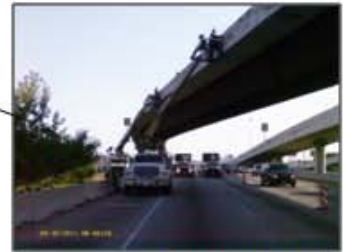
Connecting Conduit to the Bridge
